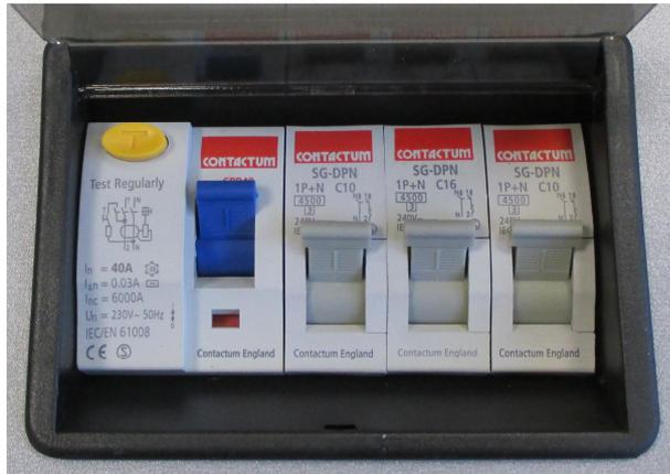
Lever type switch, far left – Residual Current Device (RCD) and main 230V on / off switch.
