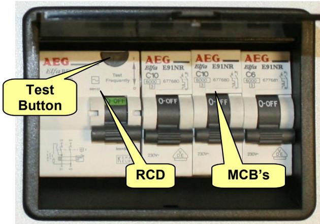
The Residual Current Device (RCD) is basically provided to protect the user from lethal electric shock. The RCD will turn off (trip) if the current flowing in the live conductor does not fully return down the neutral conductor, i.e. some current is passing through a person down to earth or through a faulty appliance.
